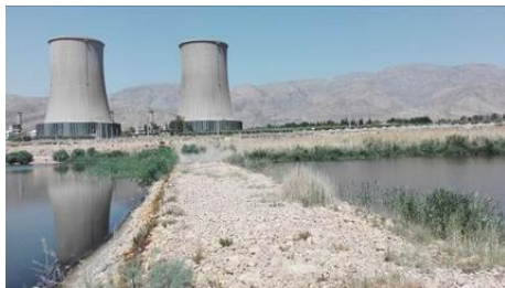
Figure 2. Sampling region at Fars combined cycle power plant.
